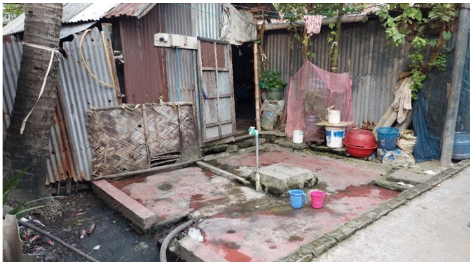
Figure 22: Water from this submersible connected pipeline is undrinkable due to odour problem in Nurani Mahalla
