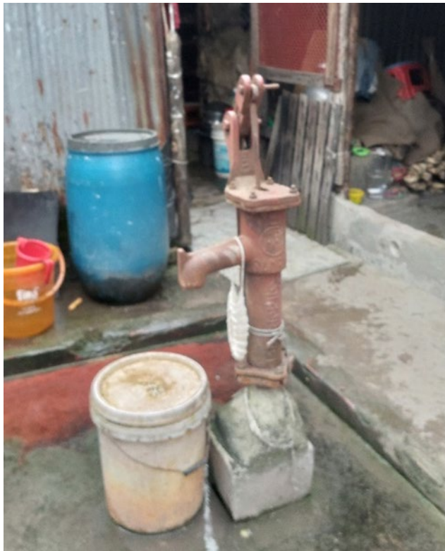
Figure 23: Nonfunctional deep tube well in Nurani Mahalla
