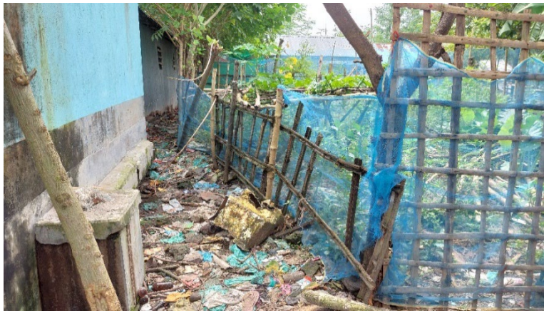
Figure 15: Outlet of human sludge is directly connected to the vegetable garden
